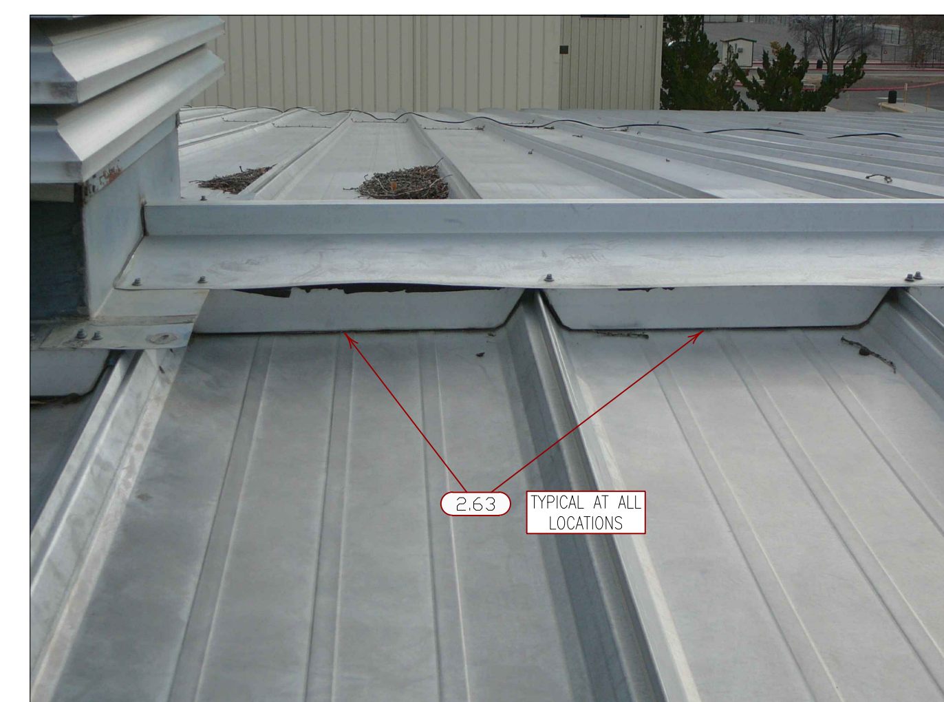
2.63 SEAL METAL CLOSURES TO THE ROOF PANELS.
