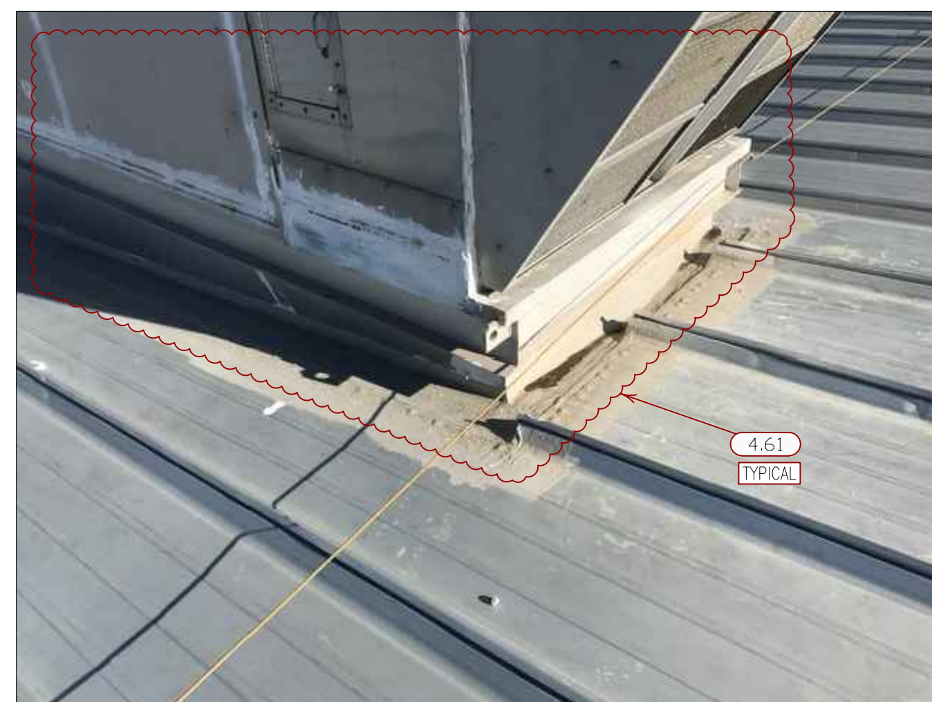
4.61 SEAL OPENINGS AT CURB FLASHING AND ROOF TOP UNIT.
