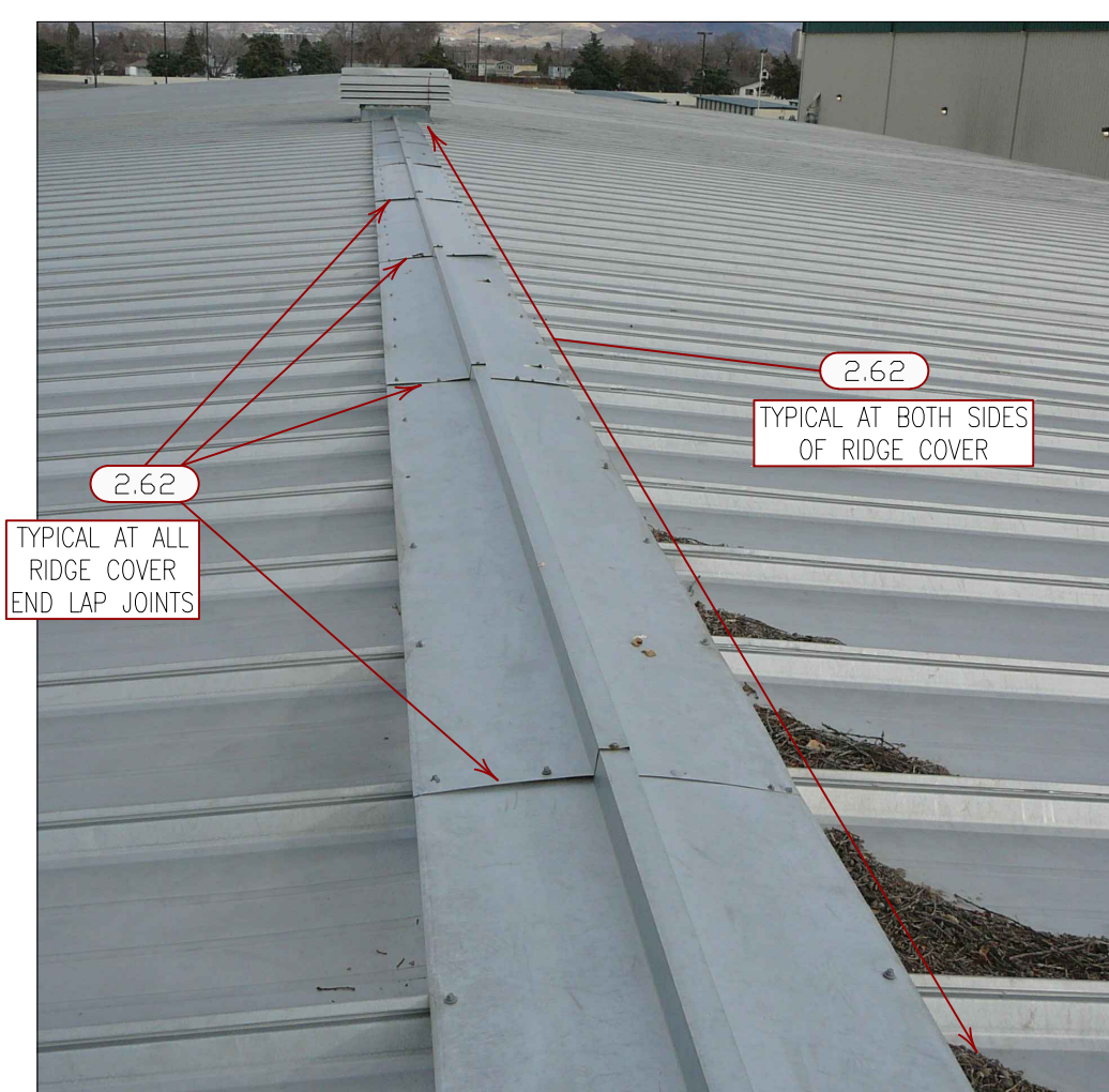
2.62 REMOVE RIDGE COVER, SEAL AND SECURE RIDGE COVER END LAP JOINTS AND TO THE METAL CLOSURES.
