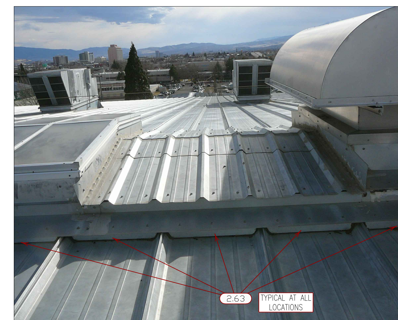
2.63 SEAL METAL CLOSURES TO THE ROOF PANELS.
