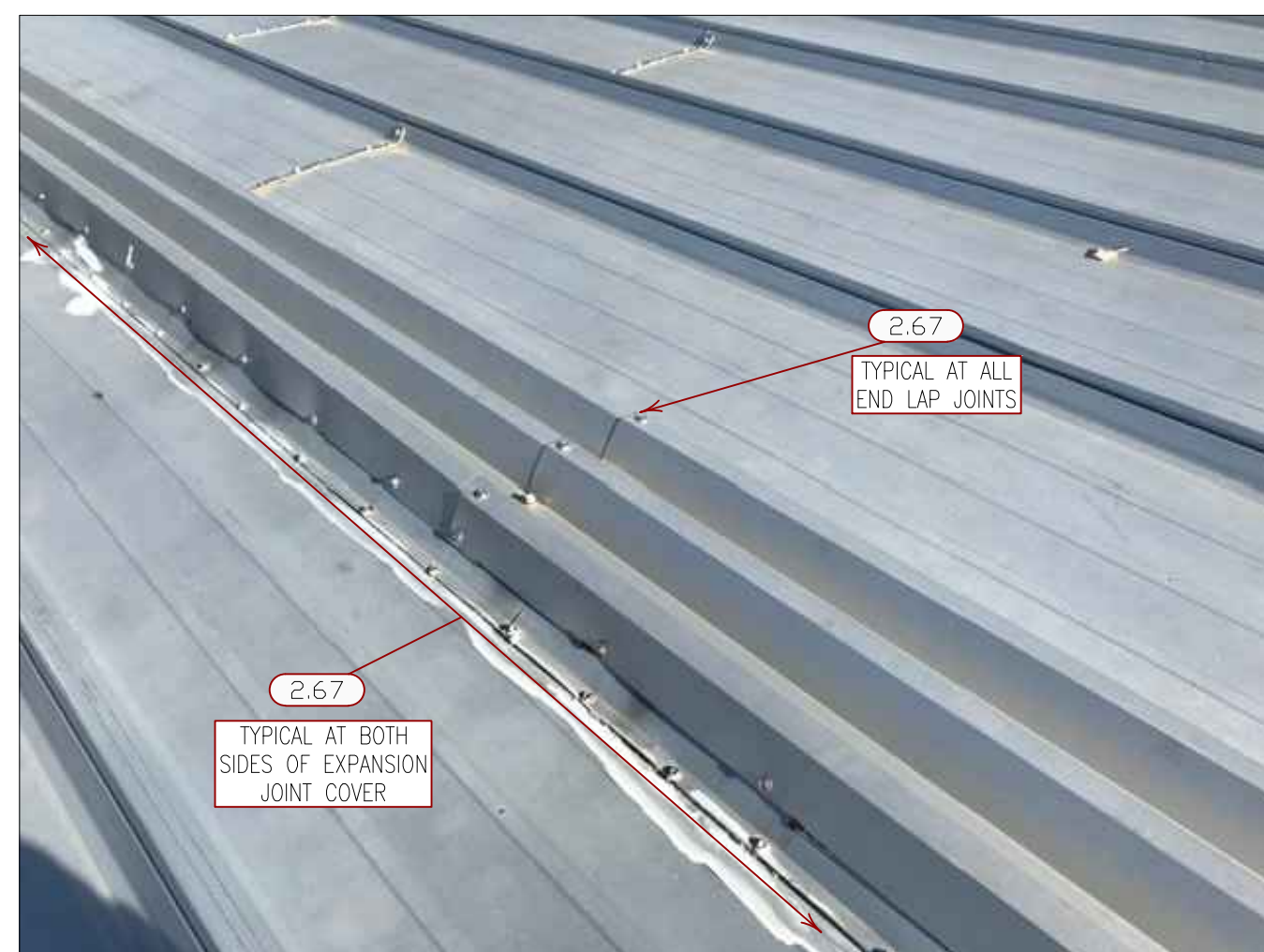
2.67 REMOVE EXPANSION JOINT COVER, SEAL AND SECURE EXPANSION JOINT COVER END LAP JOINTS AND TO THE ROOF PANELS.
