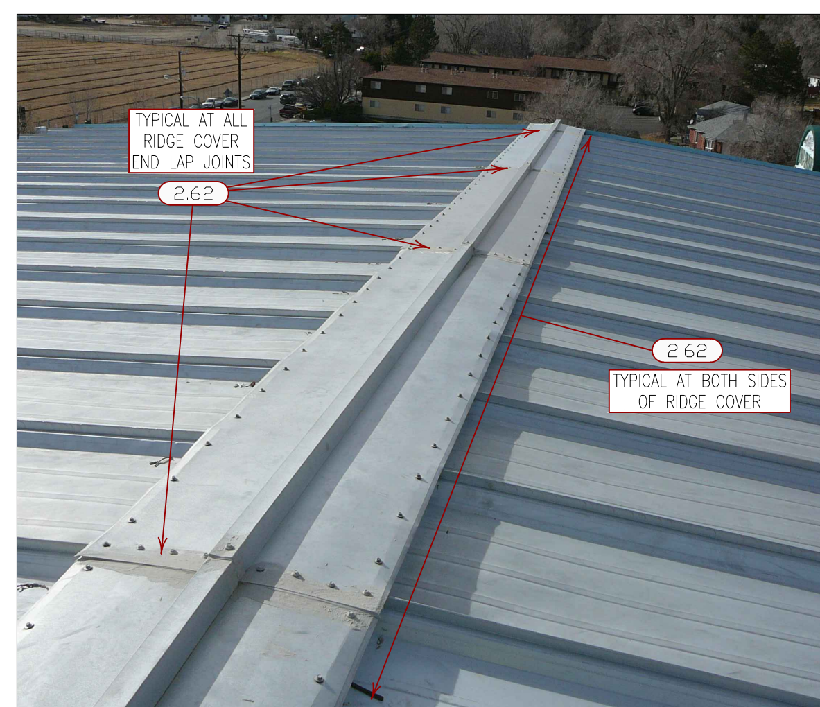
2.62 REMOVE RIDGE COVER, SEAL AND SECURE RIDGE COVER END LAP JOINTS AND TO THE METAL CLOSURES.
