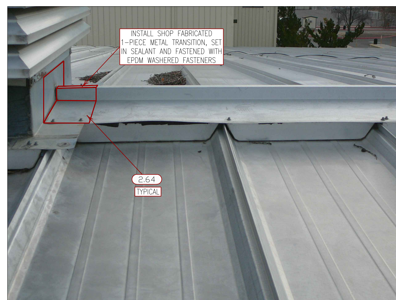
2.64 SEAL AND FLASH RIDGE COVER TO THE ROOF CURB.
